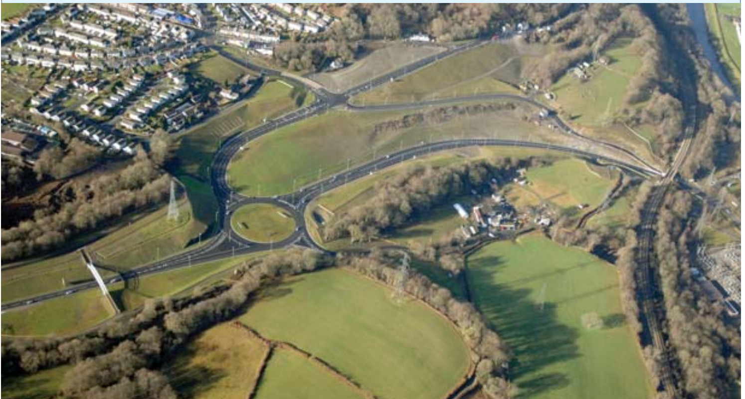
Part of the completed works at Church Village – courtesy of Costain
