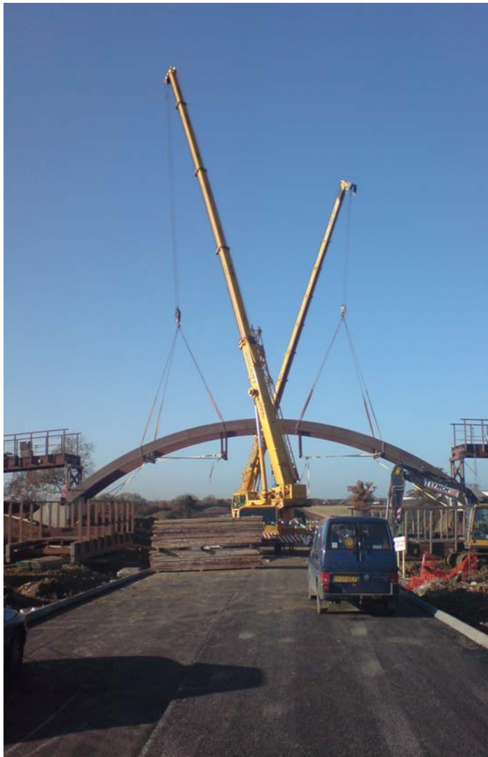
Installation of Timber Footbridge at Ridgmont Bypass
