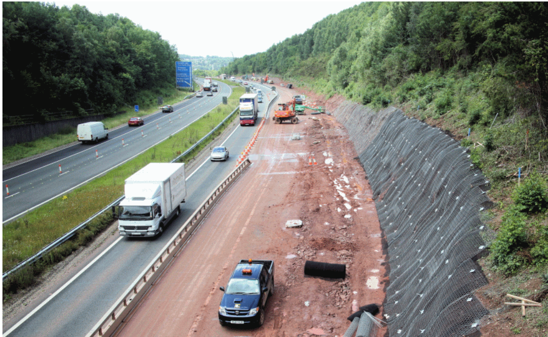
M4 Widening Junctions 29 to 32
