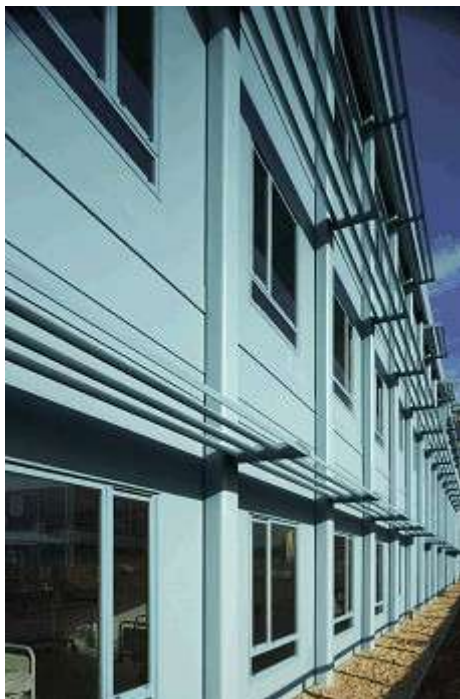
Watford General Hospital Acute Admissions Unit Courtesy of Turner & Townsend Project Management
